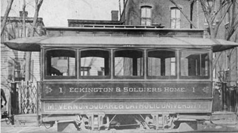
This streetcar ran up 7th Street then out New York Avenue and then to Eckington. It was the first electrified streetcar in the city—and was the only line with overhead lines.
